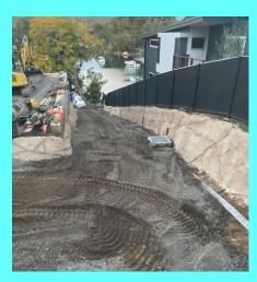
The driveway was excavated, and a lot of soil removed from the curving section of the drive to lower the incline. Then the edging was rectified by shotcreting the wall, and unlike the shotcrete we put in three years ago to stabilise the whole thing, this time we had it sculptured to look like rock.
